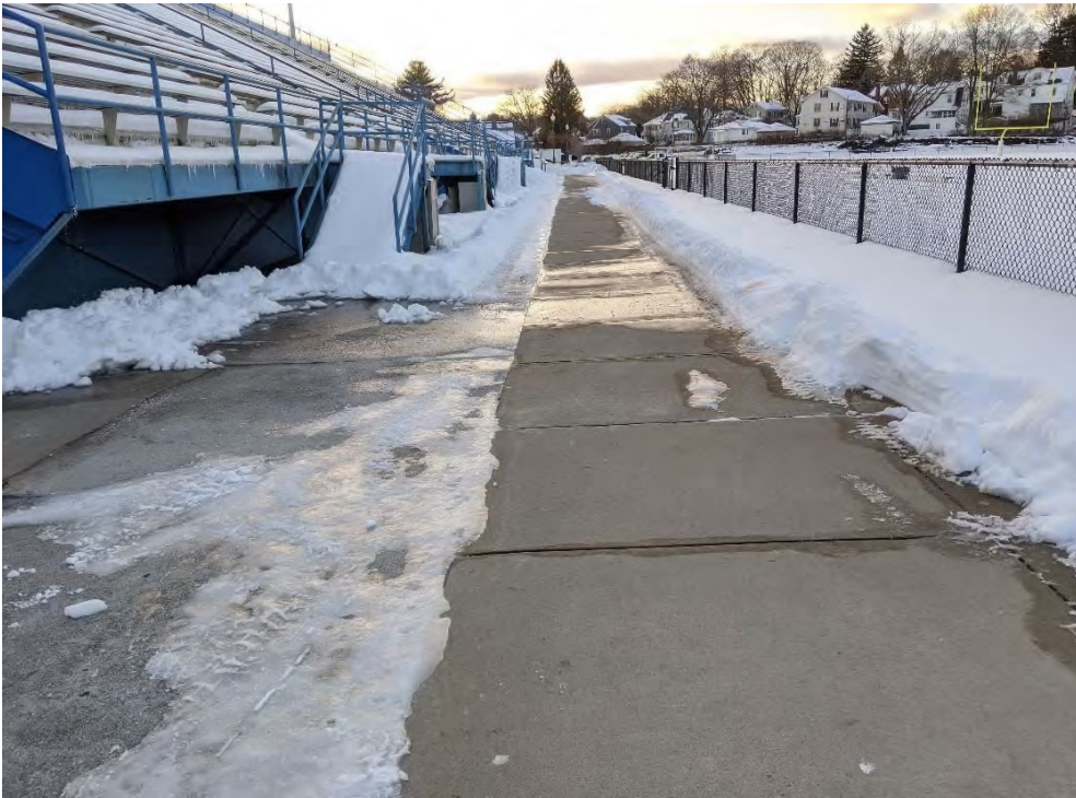
Photo No. 5: Plowed concrete walkway with no evidence of gross settlement
