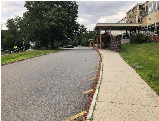
Picture 7: Pavement – Good Condition Front Access Drive / Bus Loop
