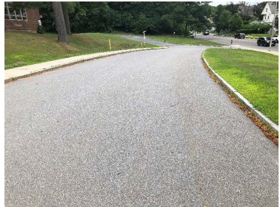
Picture 8: Pavement – Good Condition Front Access Drive / Bus Loop
