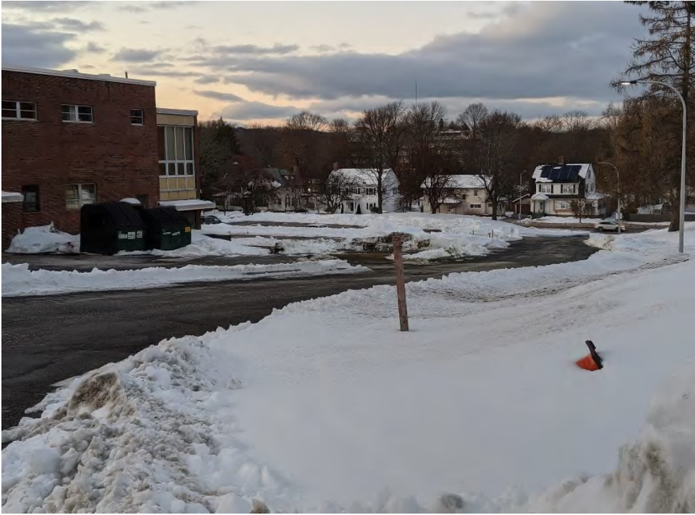
Photo No. 1: Drop in the grade from the existing parking lot to Highland Street (Looking north)
